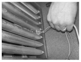
Step 16: Slide pilot assembly to back of burner rack
